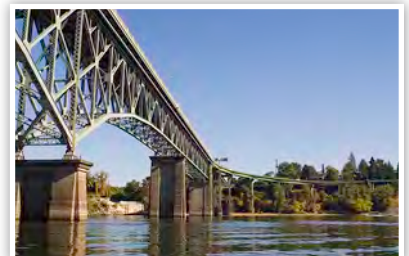
ROSS ISLAND BRIDGE
