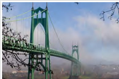
ST. JOHNS BRIDGE
