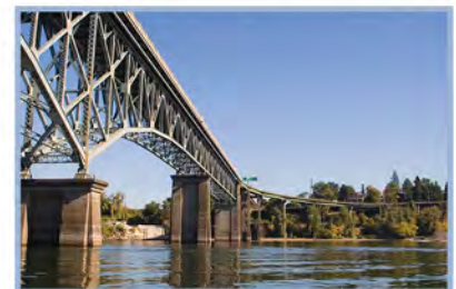
ROSS ISLAND BRIDGE
